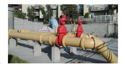
With a design capacity of 26 million gallons per day (MGD), MAPS is a critical component of the Coastal Interceptor Sewer (CIS), which moves wastewater along the coast from northern Los Angeles through Santa Monica and eventually to the Hyperion Treatment Plant in El Segundo for treatment and disposal. MAPS has been in operation since 2001 and requires improvements including pumps and electrical equipment.
