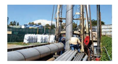
recharge well, SM-12i, to replenish the City's groundwater aquifers or augment the raw groundwater supply. The groundwater recharge well will utilize advanced treated recycled water from the City's Sustainable Water Infrastructure Project (SWIP) for recharge or augment the City's raw groundwater supply to aid in the sustainable management of the groundwater aquifers. The project will include a concrete pad, mechanical equipment, electrical equipment, and fencing.
