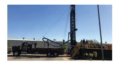
SM-11i to replenish the City's groundwater aquifers. The groundwater recharge well will utilize advanced treated recycled water from the City's Sustainable Water Infrastructure Project (SWIP) for recharge and to aid in the sustainable management of the groundwater aquifers. The groundwater recharge well will include a concrete pad, mechanical equipment, electrical equipment, and fencing.
