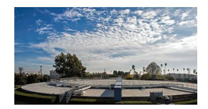
meet the water demands of the community. The four reservoirs have a combined storage volume of approximately 40 million gallons. The oldest reservoir of the four has been in service for nearly 100 years. This project will fund the needed upgrades and improvements to each reservoir that are needed to maintain reliable drinking water service for the City and to comply with recent regulatory updates.
