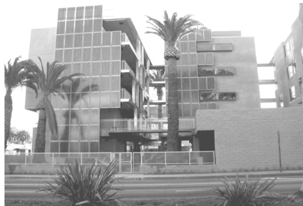
502 Colorado Housing Project
