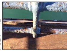
poles are also showing significant corrosion and a similar program of periodic replacement will be established.
